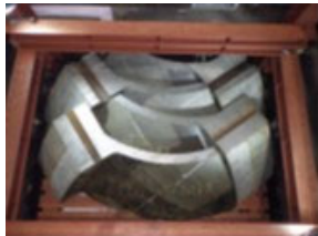
After cutting RPV Head
