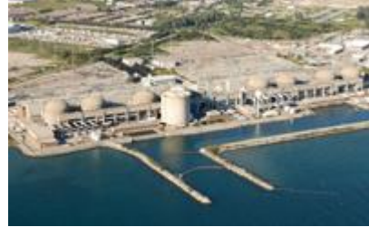
Pickering (OPG WWW site)
