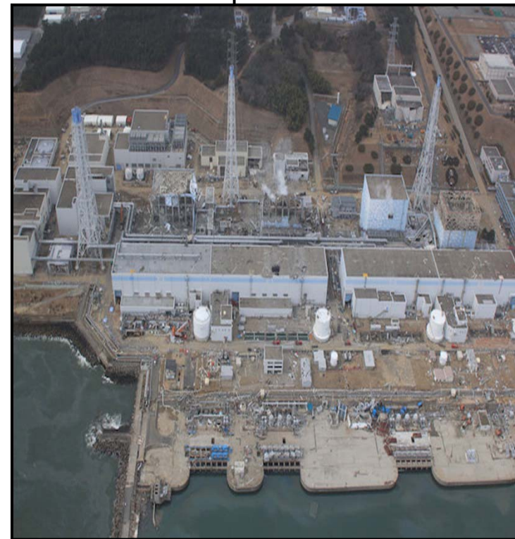
After the Earthquake and Tsunamis
