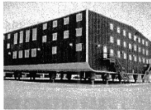
BP operations center, Prudhoe Bay, Alaska, built on pilings to resist damage from thawing permafrost.
