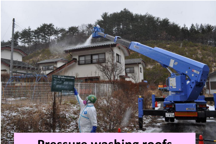
Pressure washing roofs
