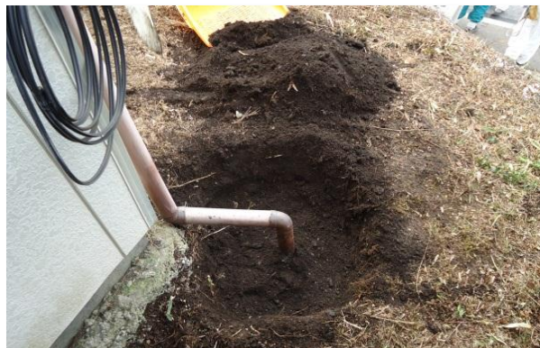
Removing drainage hotspots
