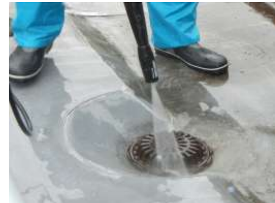
Cleaning by high-pressured water
