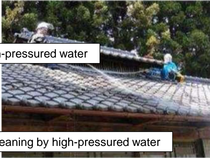
Decontamination (Back of rainwater pipe) Before: 40-50 kcpm After: less than 10kcpm
