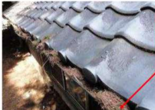
Decontamination (Back of rainwater pipe) Before: 40-50 kcpm After: less than 10kcpm
